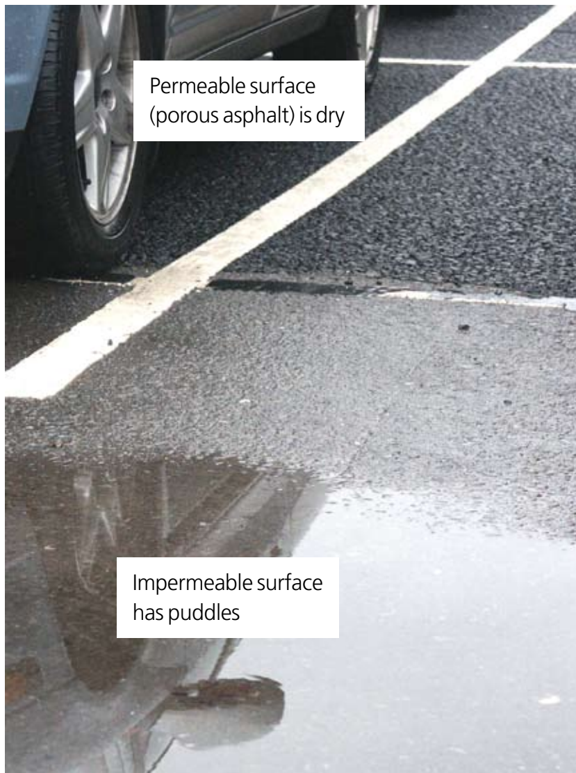
Permeable and impermeable surfaces after rainfall
